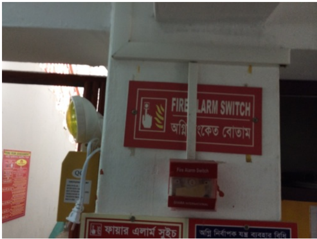
Fire alarm switch
