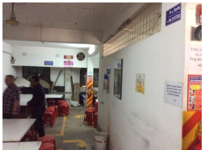
Boiler room open to floor
