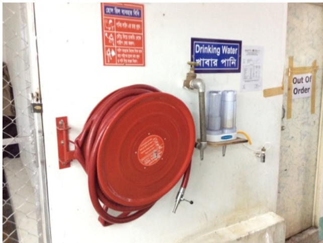
Example of fire hose
