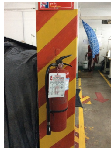
Sample of Fire Extinguishers
