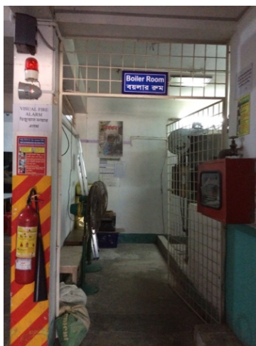
Boiler room open to floor
