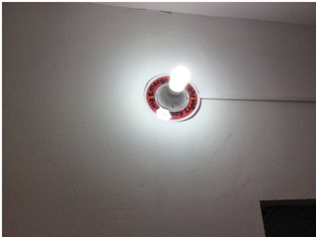
Sample of emergency light.
