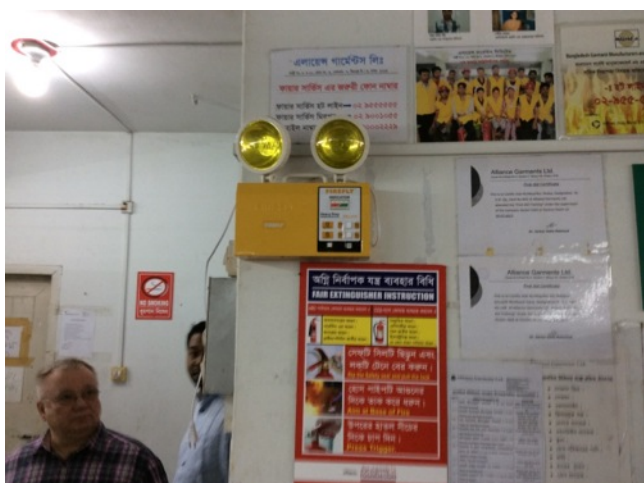
Sample of emergency light
