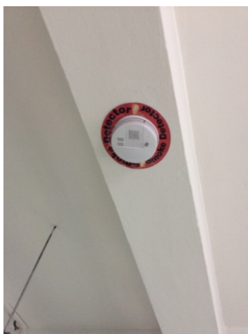
Single station smoke alarms
